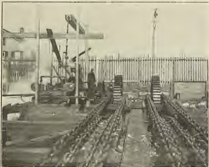
VIEW OF MACHINERY AND HAULING CHAINS—FORWARD END.
